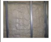
Insulation at rafter line (Warm roof) - Sloping ceilings/Flat roof
